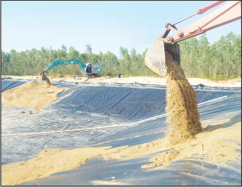
Dioxin-contaminated soils and pond sediments being placed in a passive landfill at Phu Cat Airport, March 2012. The project was completed on August 18, 2012. Courtesy of Le Ke Son
