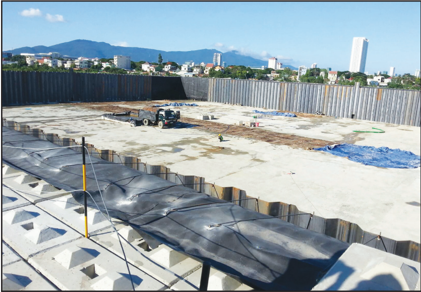
Containment structure being readied to treat dioxin-contaminated soil, Da Nang Airport, May 2013. Courtesy of Le Ke Son
