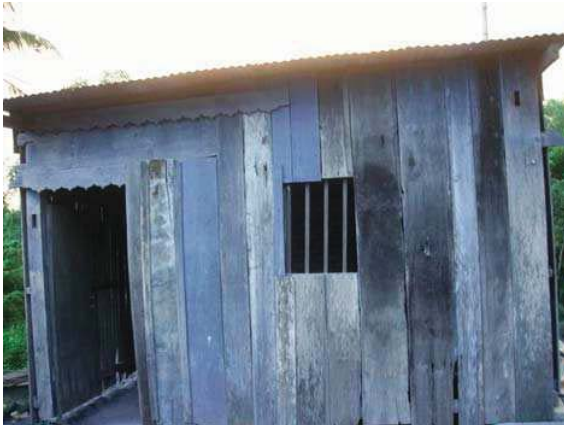
A house of PWD made from wood with metal roofing
